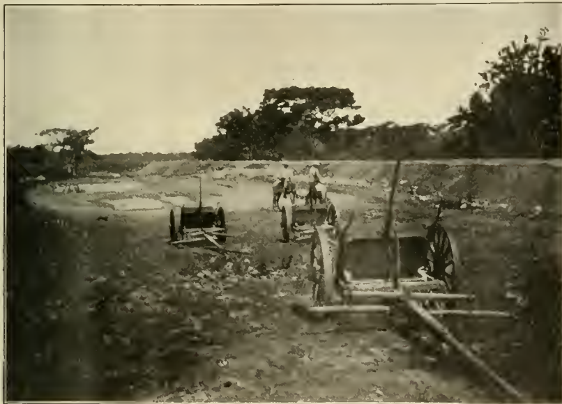
SCRAPER WORK ON THE WESTERN DIVISION.
